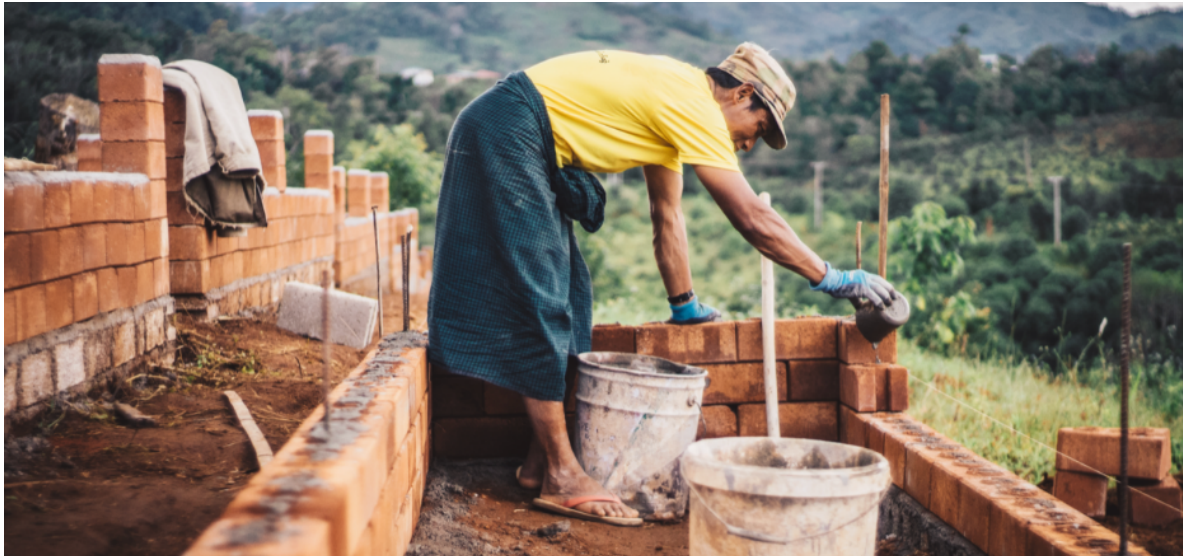
Mason building the base of a bunk bed unit, using compressed earth blocks.
